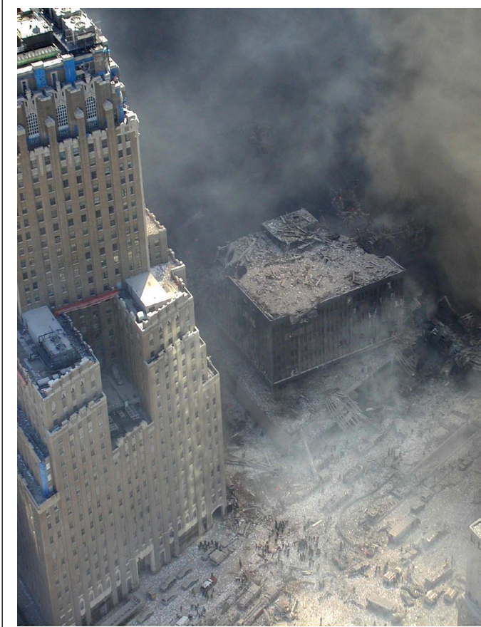
Figure 30. Looking southeast toward WTC6, across the West Street and Vesey Street intersection.
