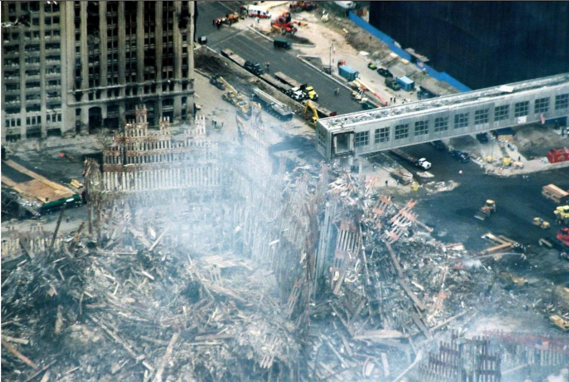
Figure 26. Most of WTC3 disappeared during the destruction of WTC1. The pedestrian walkway over the West Side Highway was connected to something that is no longer there. The remains of WTC2 can be seen near the center of the photo and the remains of WTC1 are partly visible in the lower right corner.
