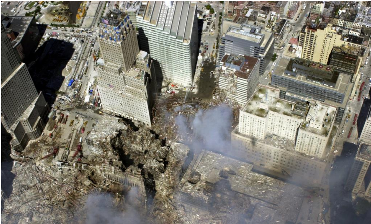
Figure 22. This photo highlights the depth of the hole in WTC6. The "smoke" or pulverized dust from debris appears to have diminished in comparison to Figure 20. While there is abundance of aluminum cladding on the roofs of buildings 5 and 6, there is little or none in the holes.
