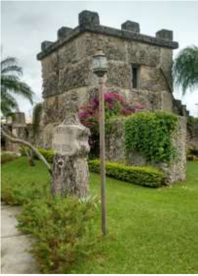
The Tower – Ed's living quarters
