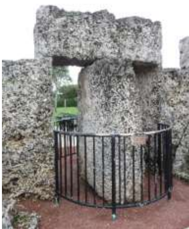
9-ton rock gate – originally span freely
