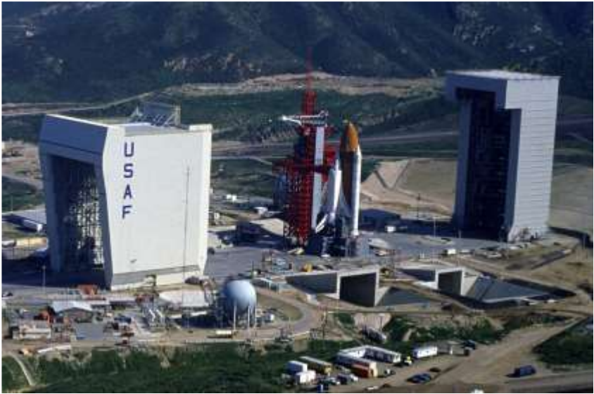
Air Force Base Space Launch Complex 6 in February 1985. 411 The space shuttle Enterprise, mated to an external tank and solid rocket boosters, is resting on the launch mount.
