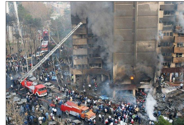
Figure 23: A C-130, about half the weight of a Boeing 767, hit this 10-story apartment building at approximately the 8 th floor in Tehran last December and crumpled outside, throwing debris around and spilling burning jet fuel over the impact wall and inside the building.
