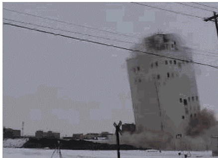
Figure 5(a): Failed demolition in South Dakota. (mov) (wmv)
