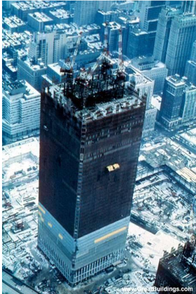
Figure 3(b): Loss of a chunk (sizable section) out of this tower would be inconsequential.
