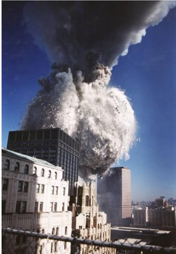
Figure 9: The tower is being peeled downward. Dark explosions shoot up, while white ones explode outward. Above the white explosions the building has vanished while the lower part awaits termination.
